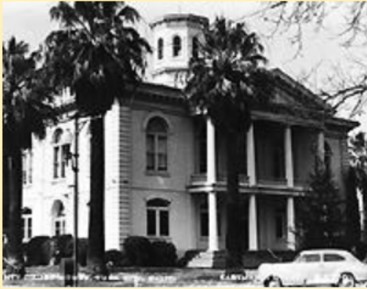
Sutter County Courthouse Completed 1900
